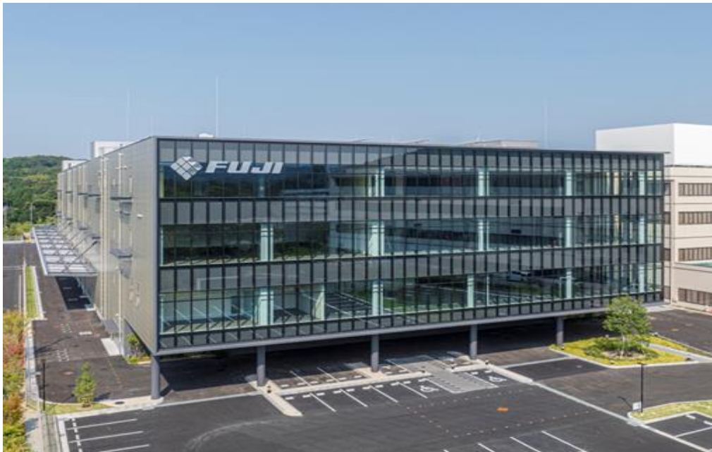
New Okazaki Plant building
