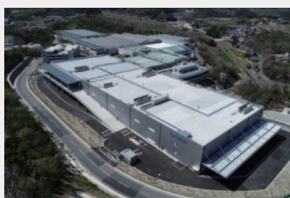
New production building in Toyota Plant
